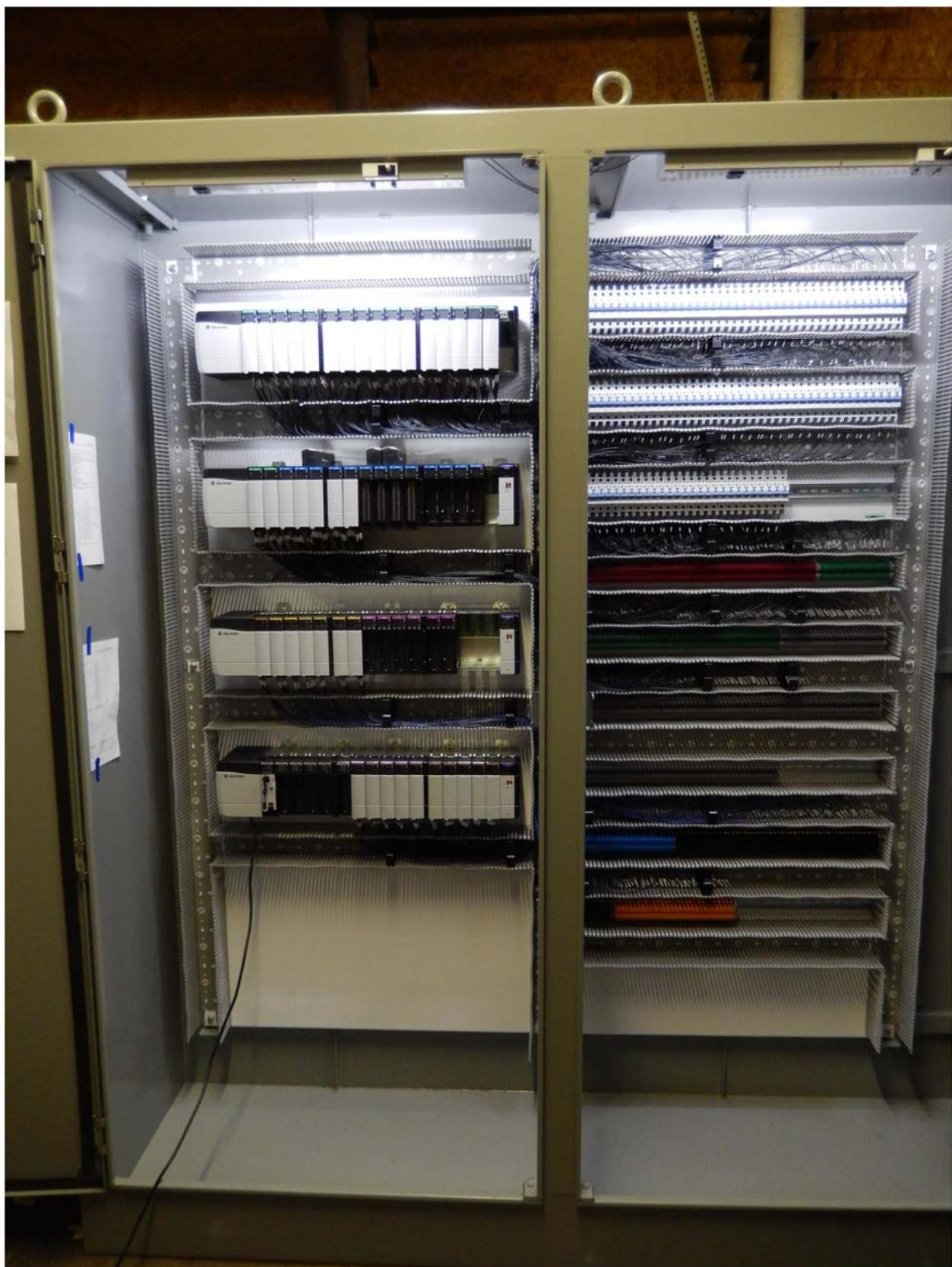
High Output LED lights (low energy does not add much heat to cabinet when on) (lights turn off automatically when door closes)
