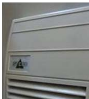
IP55 rated Air Filter present on side of the enclosure
