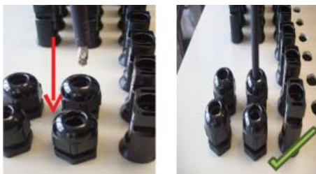
Connecting PV strings into glands
