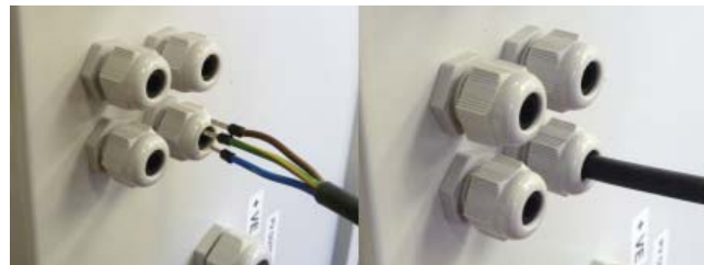
Connecting ancillary cables into glands
