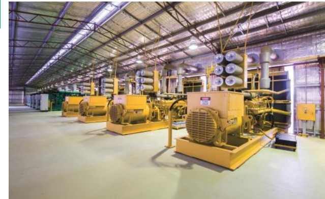
Pacific Energy engines retro-fitted with Bowman TurboGens™
